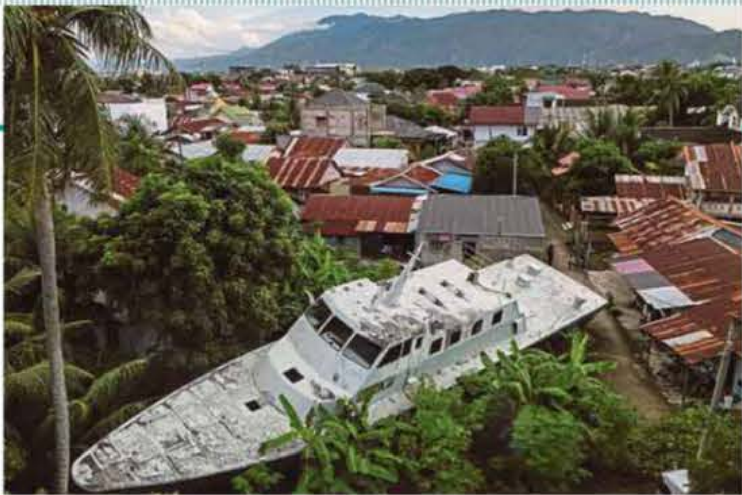
A drone view of a coast guard ship that was carried about 5km inland to the city centre of Banda Aceh during the 2004 Indian Ocean tsunami. REUTERS PIC
