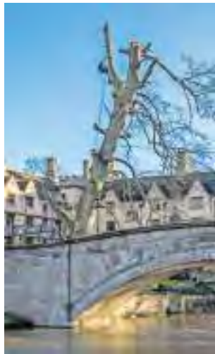
It was felled before it could fall and demolish the bridge
