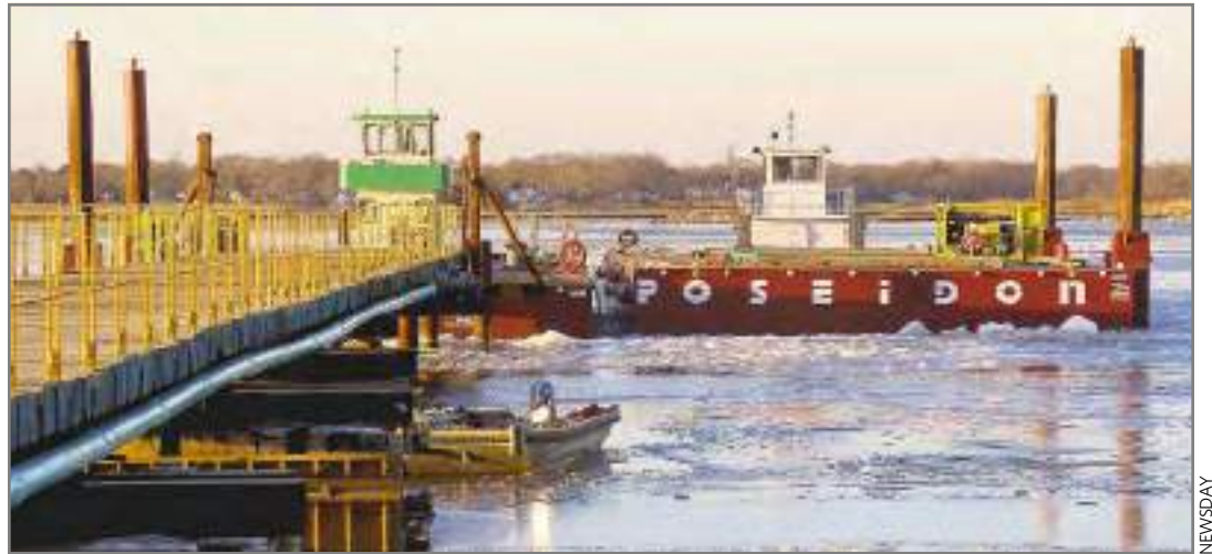
Temporary pier facilities for Sunrise Wind equipment transport barges are seen at Smith Point.
